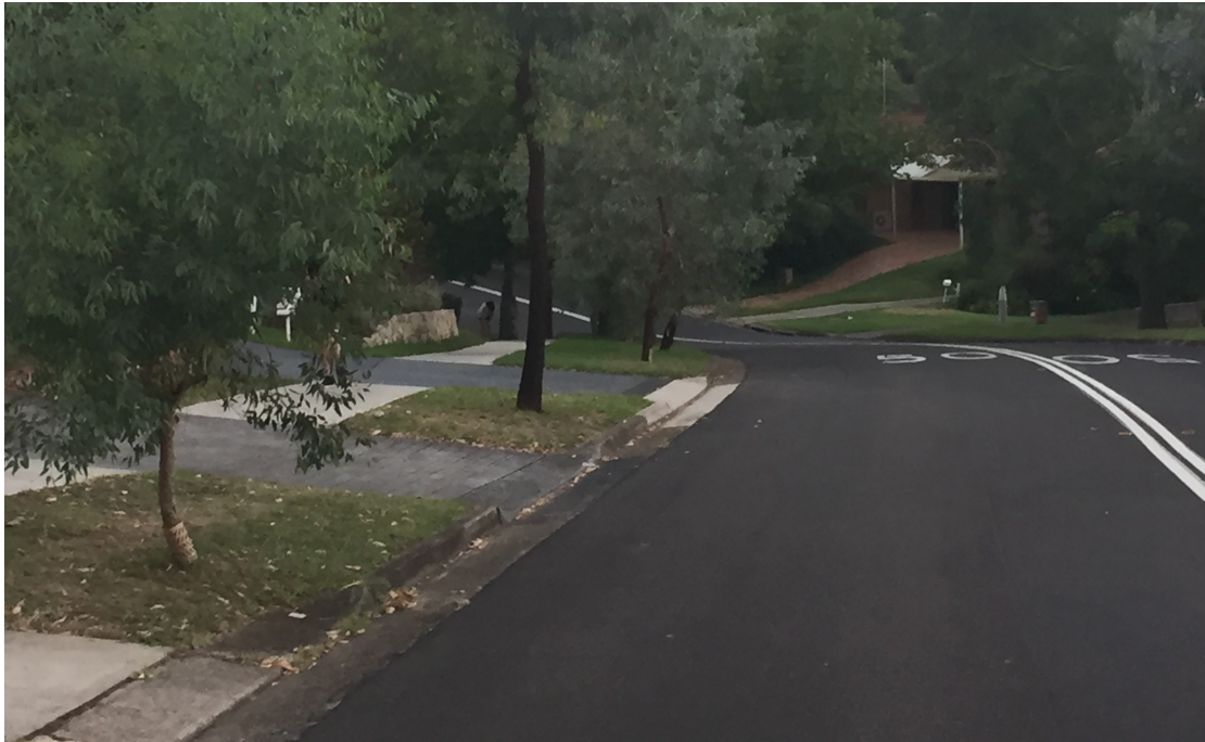
Approach along Middleton Avenue, highlighting blind spot area for drivers coming out of the proposed Cadman Crescent connection. This new road will not be visible to drivers coming along Middleton Avenue until they are only metres away from the new road.
